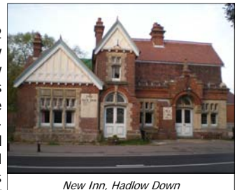
New Inn, Hadlow Down
